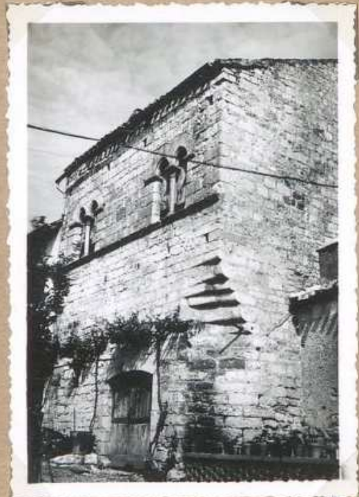
7464 M on Raynaly. facade SE
