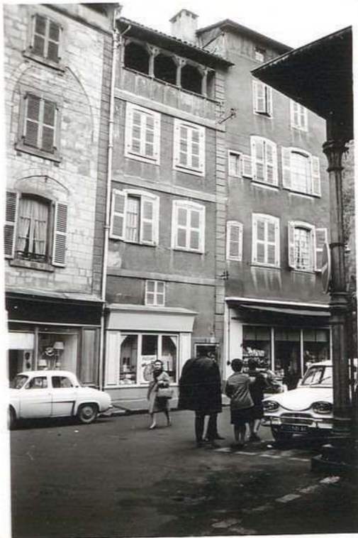
12.662 Immeuble Rogues 13, place Carnot
