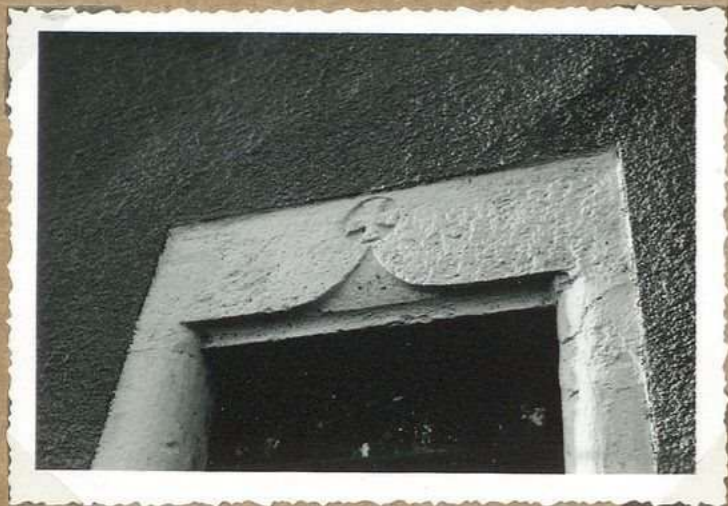
8032 M me Gaberstättle .S. Linteau accolade
