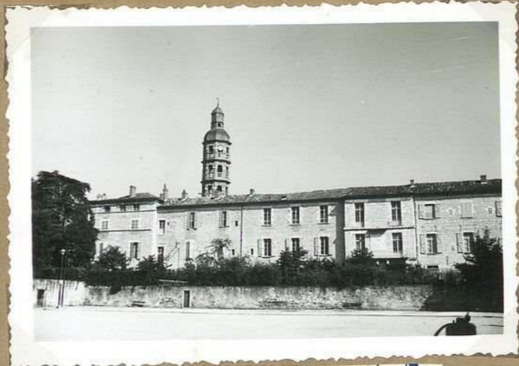
8584. Lycée Gambetta facade S.
