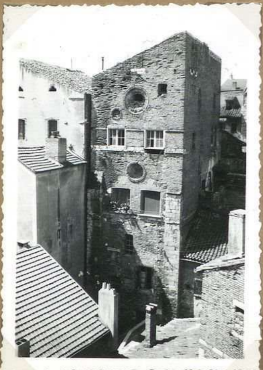
8455. 2. Rue du Four St Catherine, facade N.
