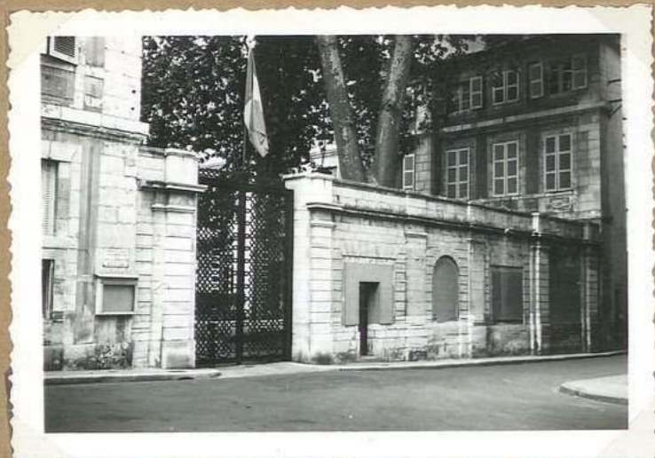
8680. Prefecture. facade S.
