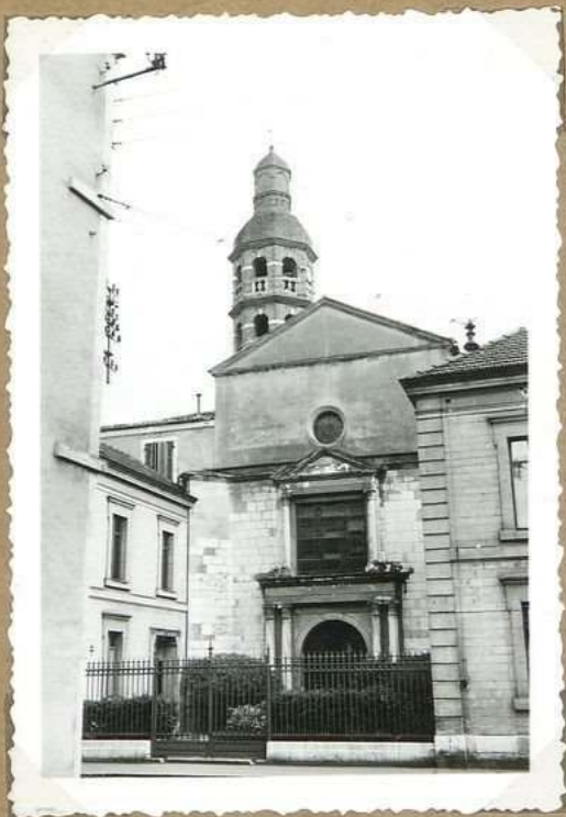
8595 Lycée Gambetta Chapelle - facade N ensemble
