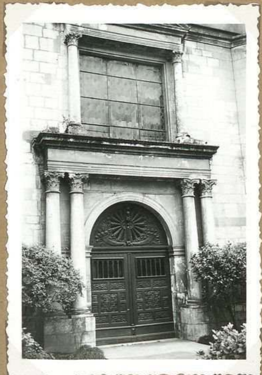
8585. Lycée Gambetta La Chapelle, facade N
