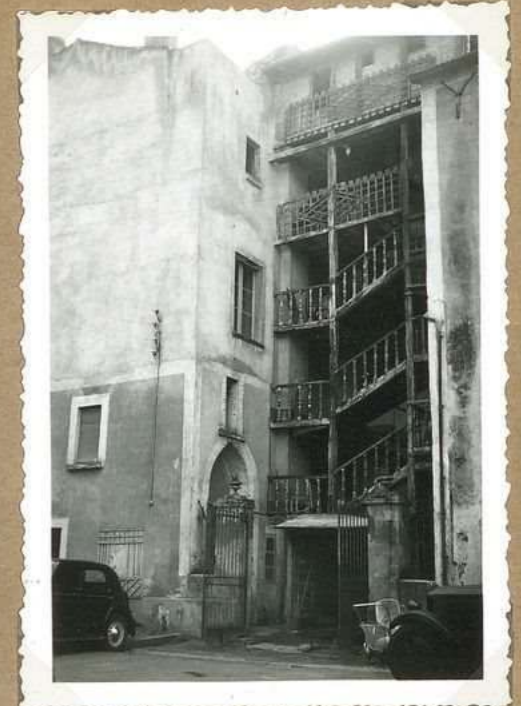
8256. Place St. Priest Escalier bois
