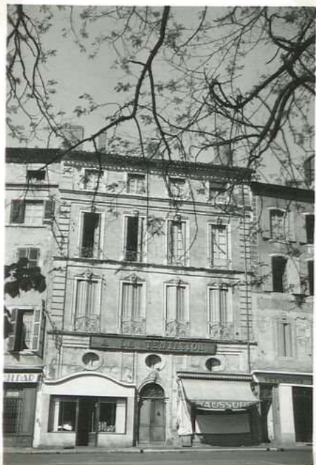
8317. 8-Place J. Chapou Ensemble facade
